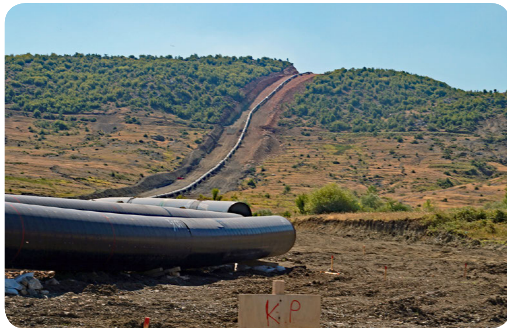
Construction of TAP pipeline in Albania
